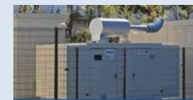
Emergency power generator
