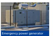
The facilities are equipped with emergency power generators that can operate for up to 72 hours for BCP response, including ensuring safety in the facility in the event of a power outage.
