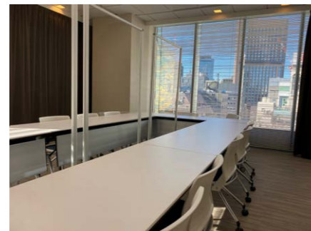
Installation of partitions in conference rooms
