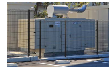
Emergency power generator
