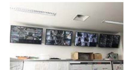
Remote monitoring using ITV
